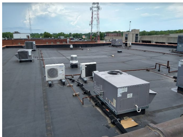
Current state of BRITE Labs Roof
